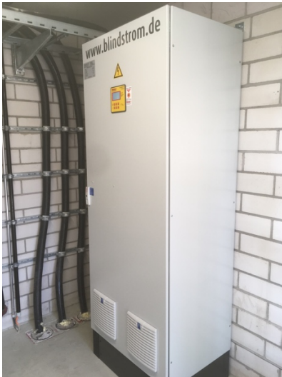
10 Reactive current compensation system
