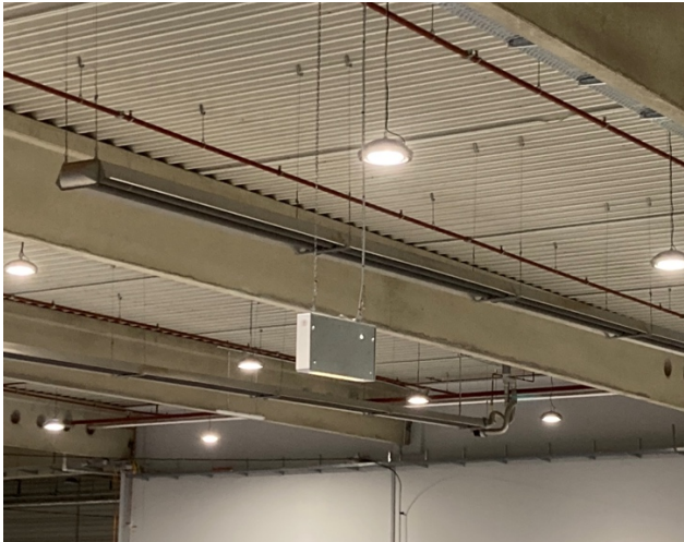
8 - Gas radiant heater
